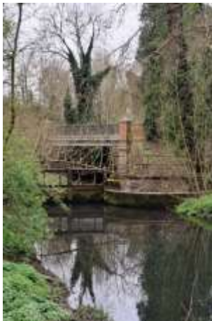
Weir across the River Beane
