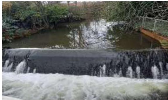
Thornton Street Weir
