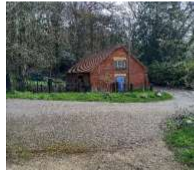
Molewood Pumping Station
