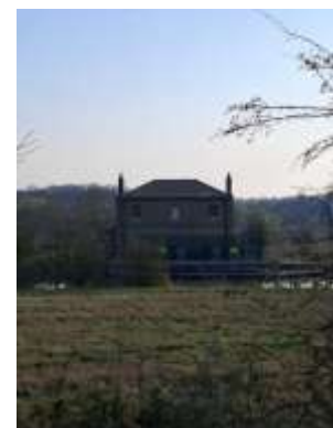
The New Gauge House
