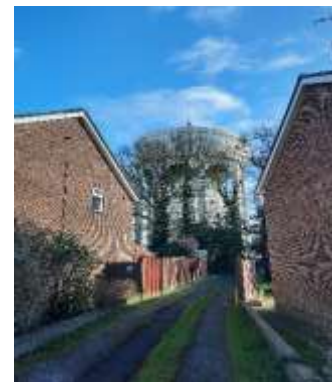
Bengo Water Tower
