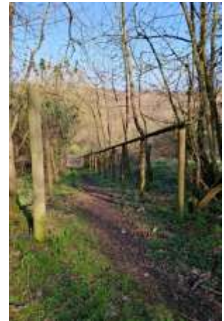
Track with handrail
