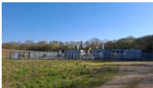
Brazier Generation Station
