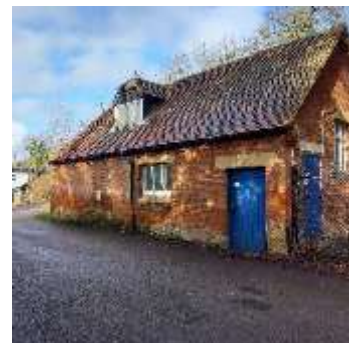
Molewood Road Pumping Station
