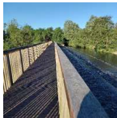
Hertford Basin Weir
