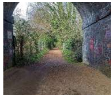
Railway tunnel on Footpath 93
