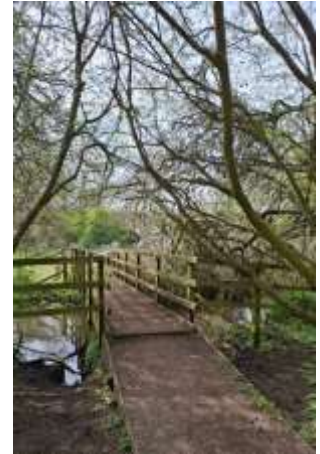
Bridge leading to the railway arch
